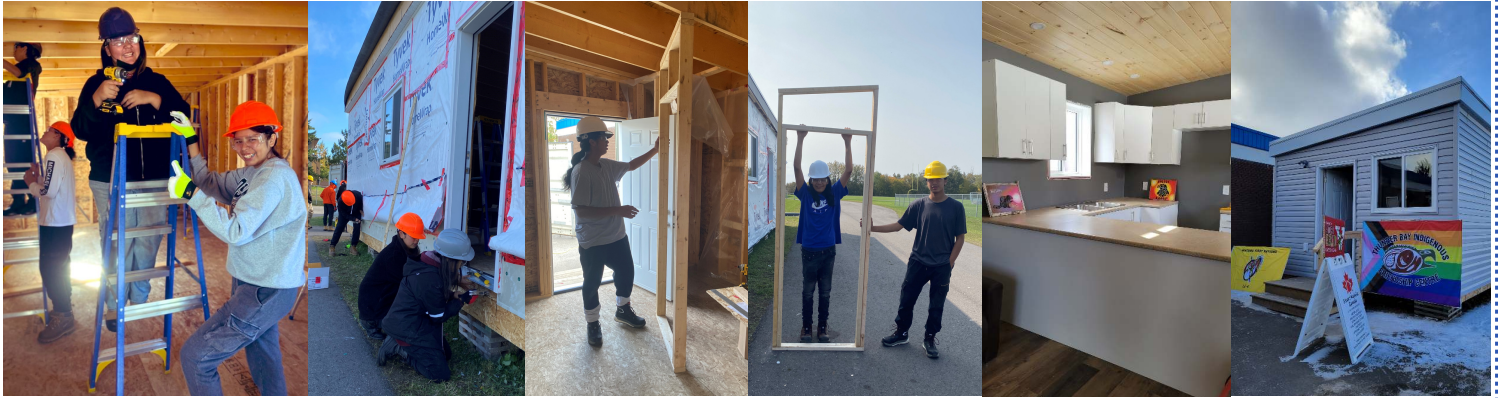
Pictured: Students working on the tiny homes project at different stages.
