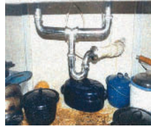
Look for gaps where the water pipes come into your house
