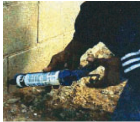
Seal holes with steel wool and caulk
